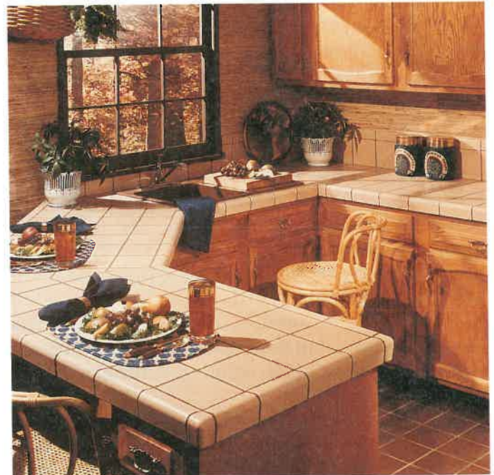
Figure 15-3. Ceramic tile provides an attractive and durable surface for this kitchen counter. (Mid-West Tile)
