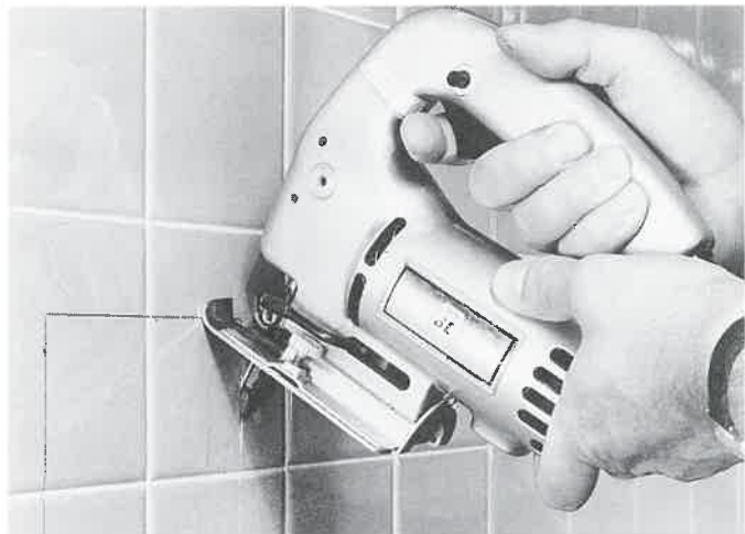
Figure 15-41. Sawing tile. A—Cut curves with a carbide blade hacksaw. B—Cut holes in tile with a saber saw. (Remington Arms Co.)
