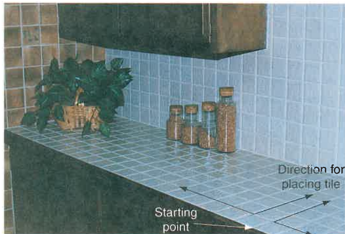
Figure 15-37. A one edge tile layout begins at the front edge. This type of layout is common for countertops.
