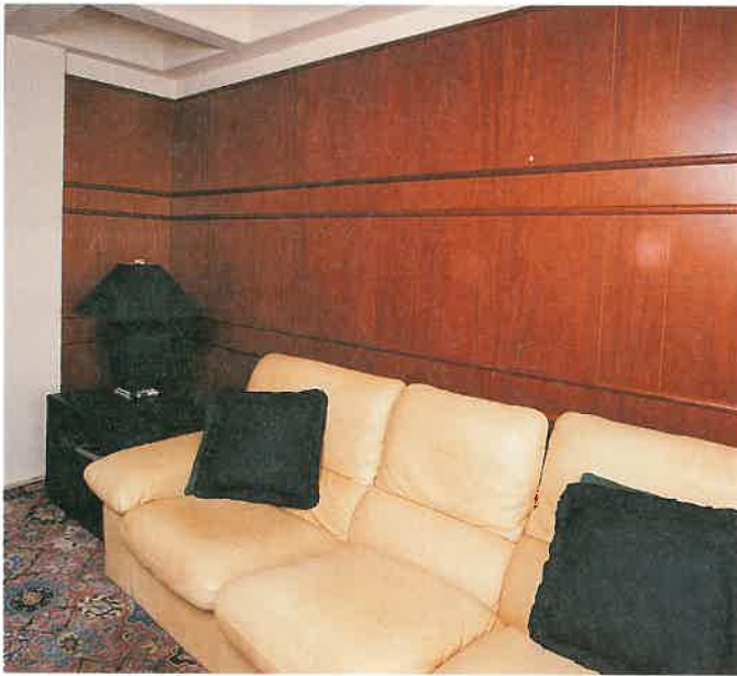
Figure 14-2. The walls of this residential study are paneled with MDF covered with mahogany wood veneer. (Chuck Davis Cabinets)
