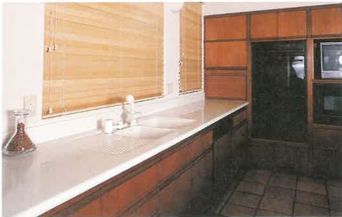
Figure 15-33. Solid surface material often replaces laminates for countertops. Solid surface material can be cut, drilled, and shaped with carbide tipped woodworking tools. (Chuck Davis Cabinets)
