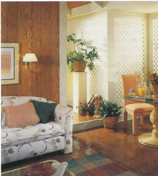
Figure 13-17. Prefinished paneling is used for wall decoration. (Georgia-Pacific Corp.)
